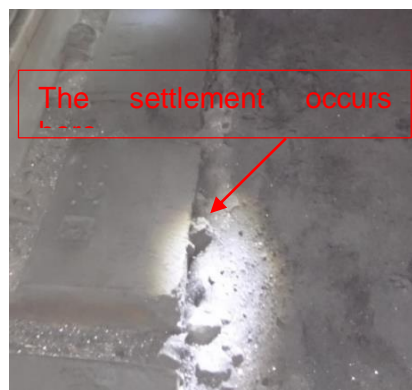
(a) Settlement of substructure
