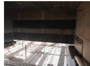
(d) Photo of steel plate pasted to cross beam
