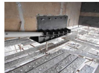
(b) Photo of external beam reinforcement of main beam
