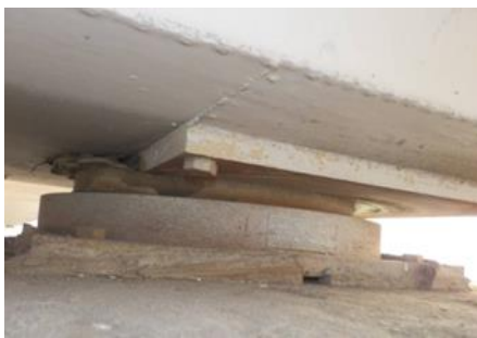
Fig. 4 – Bearing damage
