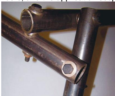
Fig. 6 - Bolted connectors
