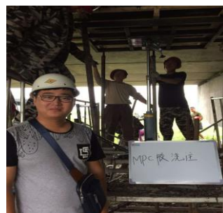
(a) Mixed the PUC material (b) Support formwork and PUC casting (c) Template removal Fig. 7 - The PUC material casting
