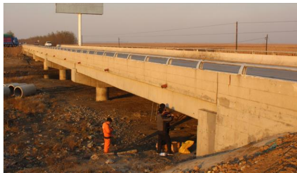
Fig. 1 - Lateral view of Piao Fa Bridge
