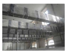
Fig. 1 – FRP sheets bonded to the external surface of RC beams
