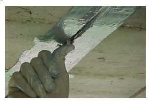
Fig. 2 – Use of FRP composites in surface grooves of a beam by the NSM method
