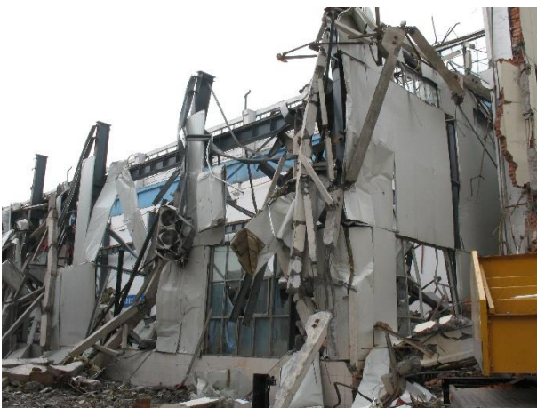
(c) Failure of steel structure industrial building
