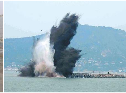
Fig.3 - Blasting compaction
