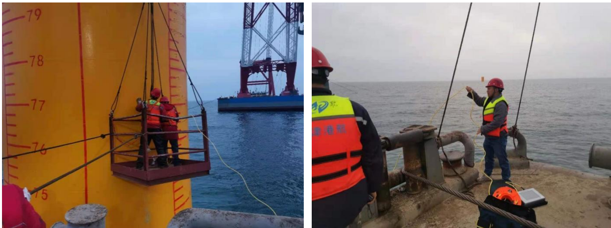
Fig. 1 – High strain detection of large-diameter monopile
