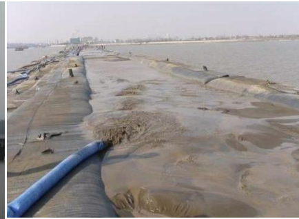
Fig.2 - Filling sand
