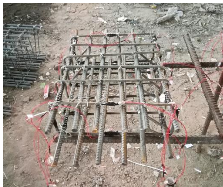
(a) Pier body reinforcement skeleton
