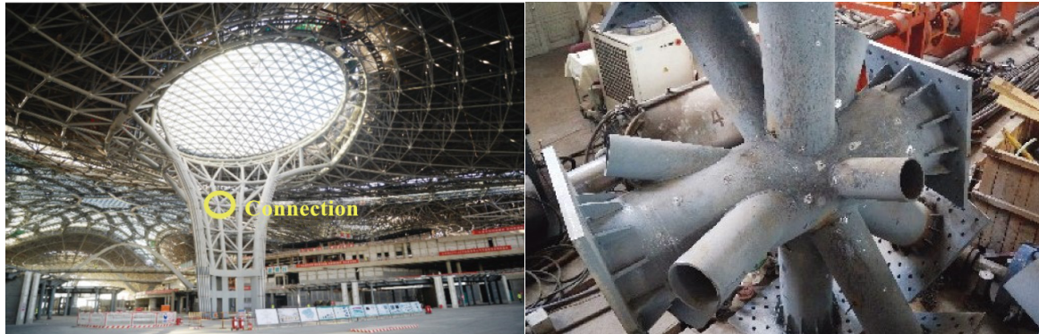
Fig. 1 - The Roof Structure of Beijing Daxing Airport Terminal
