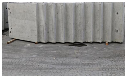
(b) Prefabricated stairs placed vertically without fixed measures
