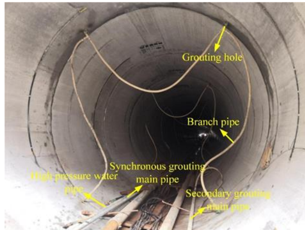
Fig. 7 – Layout of grouting pipe
