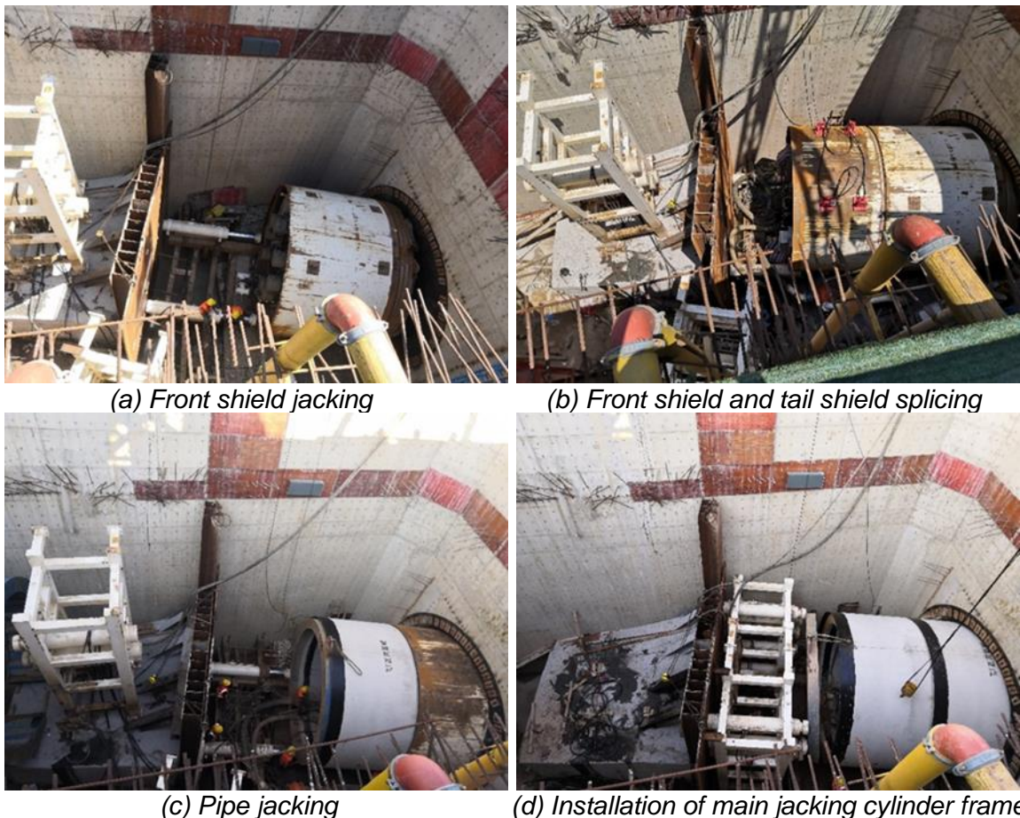
Fig. 11 – Launching step of pipe jacking
