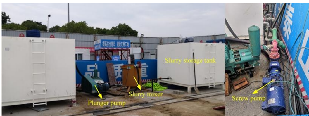
Fig. 6 – Layout of thixotropic slurry system
