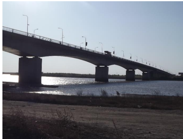
(a) Field bridge
