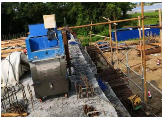
Fig. 7 - Field Diagram of Intelligent Tensioning Equipment
