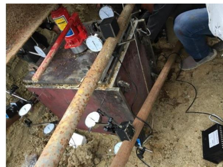
(b) On-site dial indicator installation
