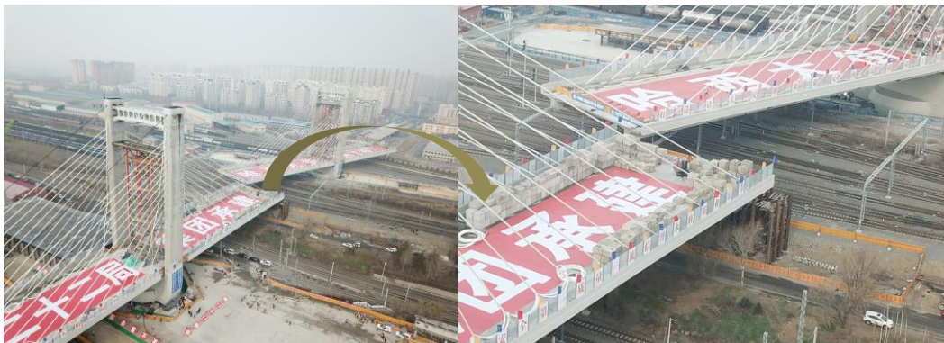
Fig. 6 - Photographs of the counterweight on site in Tower ten
