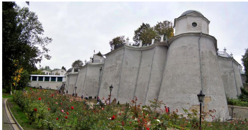
Fig. 2 – General view of the Debosquette Wall [39]
