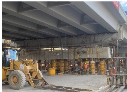
c) embracing column beam
