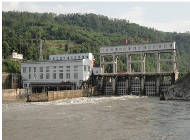
Fig. 2 – Site photos of Xinzhong Hydropower Station
