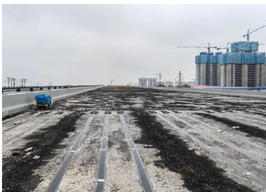
Fig. 9 - Carbon fiberboard active reinforcement diagram
