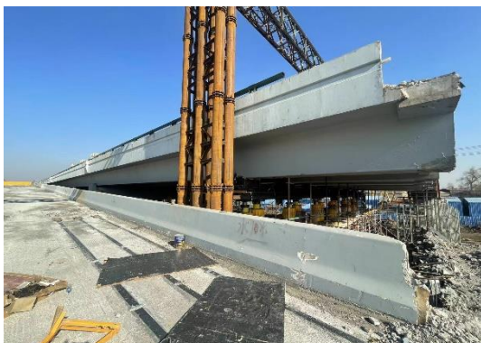
Fig. 16 - Comparison diagram of left and right bridge jacking construction
