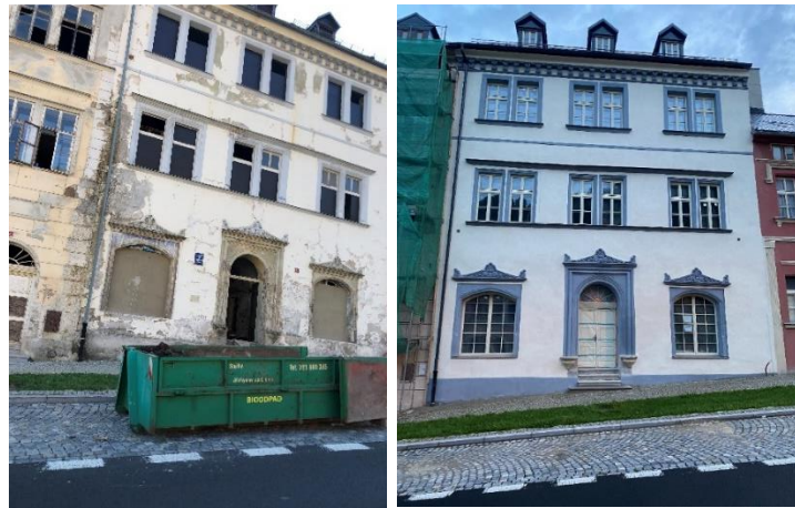
Fig.4 – The house No. 12 in Jáchymov before (left) and after reconstruction (right) in 2023.
