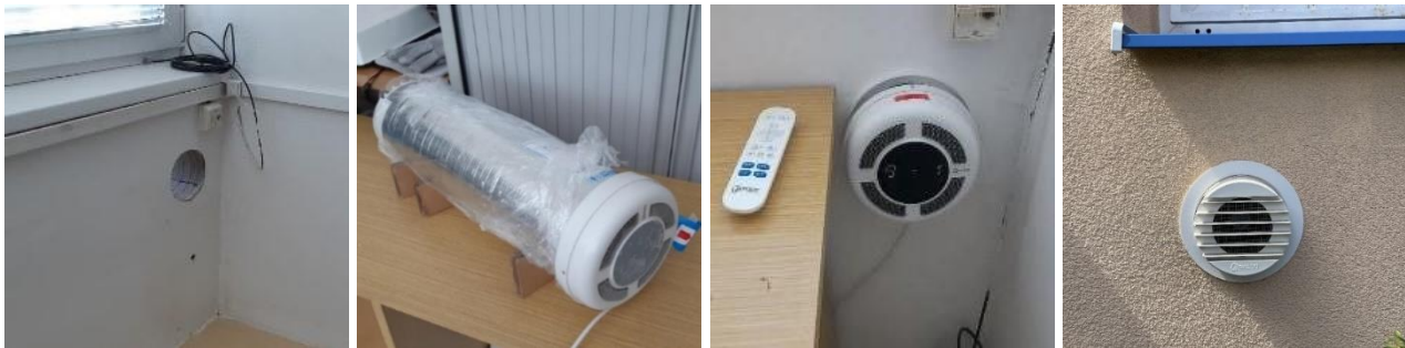
Fig. 2 – Installation of the ventilation device in the prepared place.
