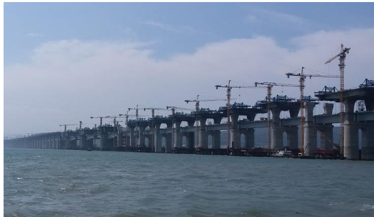
Fig. 1 – The main bridge of a dual-purpose road-rail bridge in Fujian province
