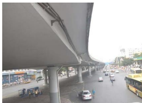
Fig. 1 – Aerial view of the elevated bridge
