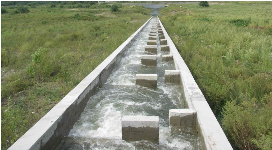
Fig.3 - Site View of the Fishway Project at Laolongkou
