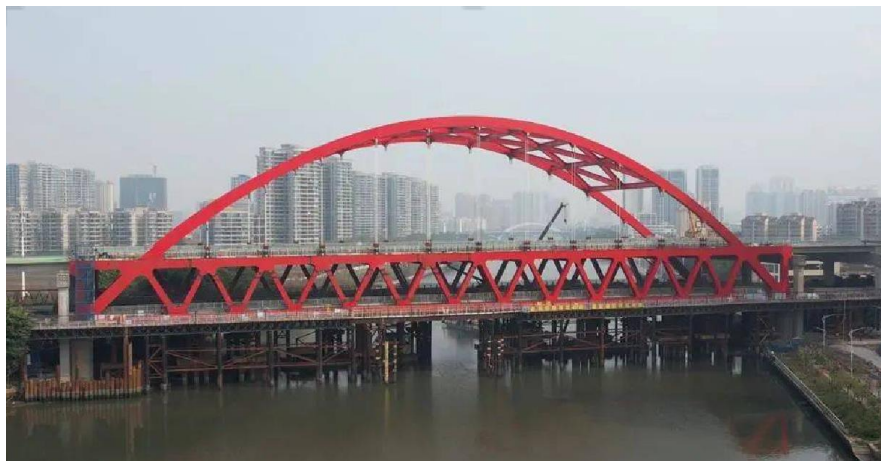
Fig. 1 – Bridge real picture
