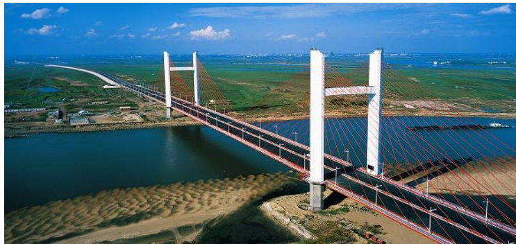
Fig. 3 - Bridge Panoramic View
