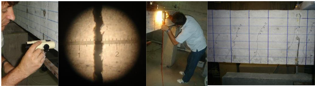
Fig. 3 - Measurement and verification of cracks [11]
