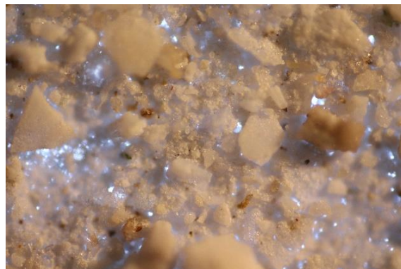
Fig. 10 – The lime efflorescence sample S1 (after crystallization)
