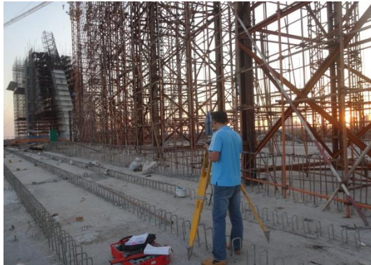
Fig.18 -Main girder elevation measurement anchor point
