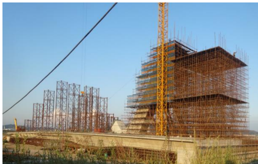
Fig. 3 - Cable tower and arch rib support
