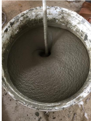
(a) Prepare foam concrete
