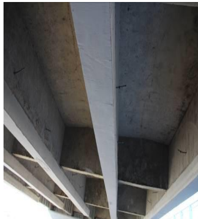
Fig .5 - Reinforcement figures of bridge two
