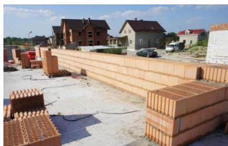
Fig. 3 – Layering of hollow ceramic blocks (Porotherm 38, Photo taken from [34])
