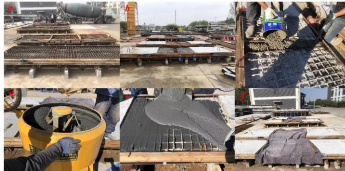
Fig. 3 – Box beam fabrication process: (a) – supporting formwork and tying reinforcement, (b) – pouring precast concrete, (c) – pouring concrete for center diaphragm, (d) – mixing UHPC, (e) – pouring UHPC, and (f) – curing after UHPC pouring
