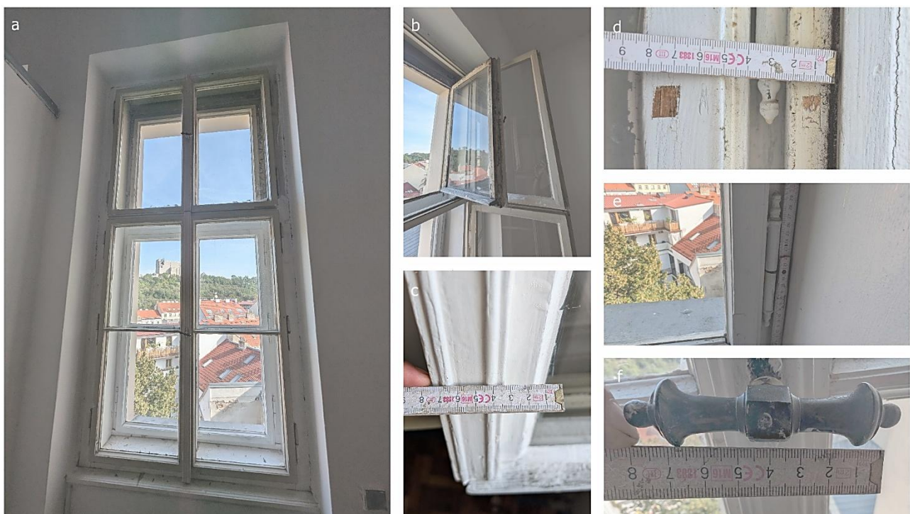
Fig. 4 - Analysed window at ZUŠ Štítného – photographic documentation a) front view of the window from the interior, b,c) detail of the profile, d,e,f) window ironmongery details.
