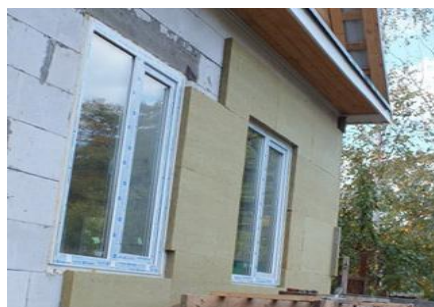
Fig. 2 – AAC façade insulated with stone-wool wall insulator (Photo taken from [33])
