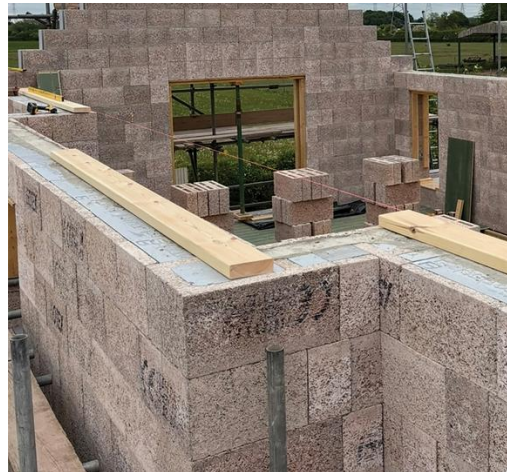
Fig. 5 – Layering of ISOTEX - ICF wood-chip cement-bonded blocks (Photo taken from [36][35][34])
